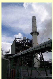
Condong Sugar Mill – NSW - 30 MW
